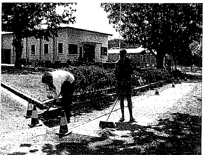
Bottom: Workers preparing area for the laying of pavers.
