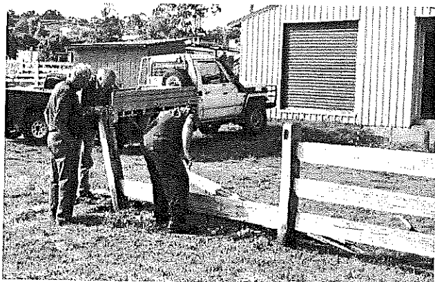
"Members of the Break O'Day Woodcraft Guild demonstrate how a post and rail fence is made".
