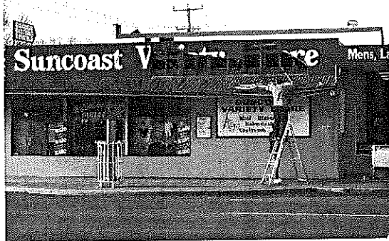
Suncoast Variety Store showing damage caused by wild weather last Thursday.
