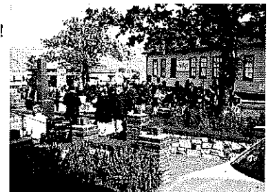
Wall which has been Demolished.
